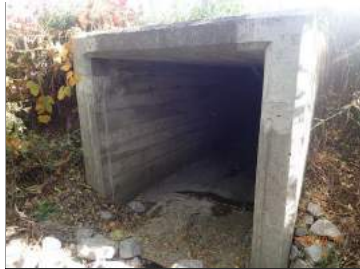
Plate 1: Colborne Creek (C1) inlet, facing south (downstream).
