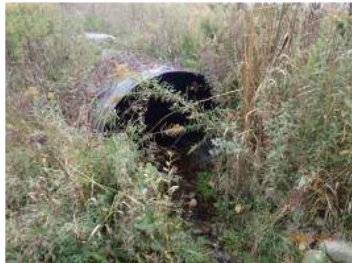
Plate 5: Unknown watercourse (C7) outlet, facing north (upstream).
