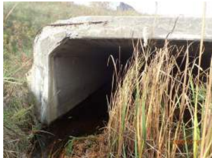
Plate 5: Bidy Creek Crossing 2 (C5) outlet, facing north (upstream).
