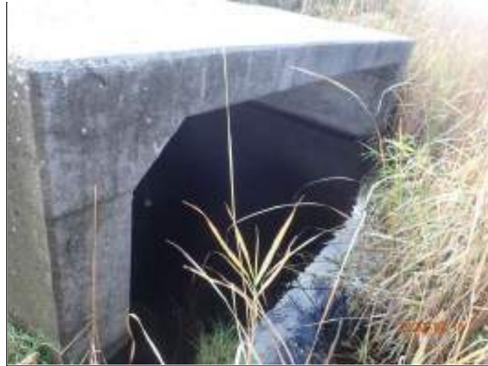
Plate 1: Bidy Creek Crossing 3 (C6) outlet, facing south (upstream).
