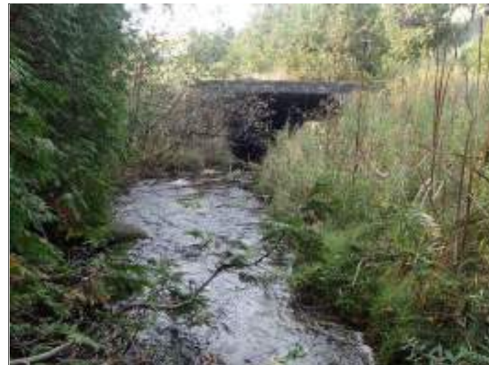
Plate 6: Biddy Creek Crossing 1 (C4) inlet, facing north (downstream).
