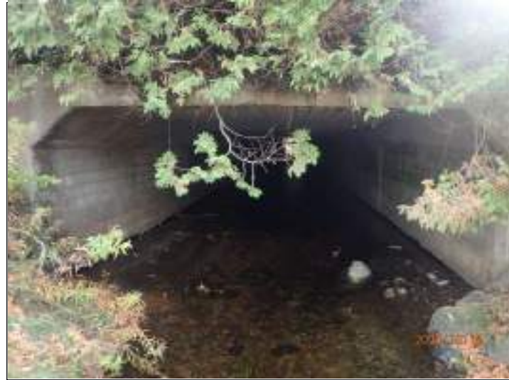
Plate 1: Bidy Creek Crossing 1 (C4) outlet, facing south (upstream).
