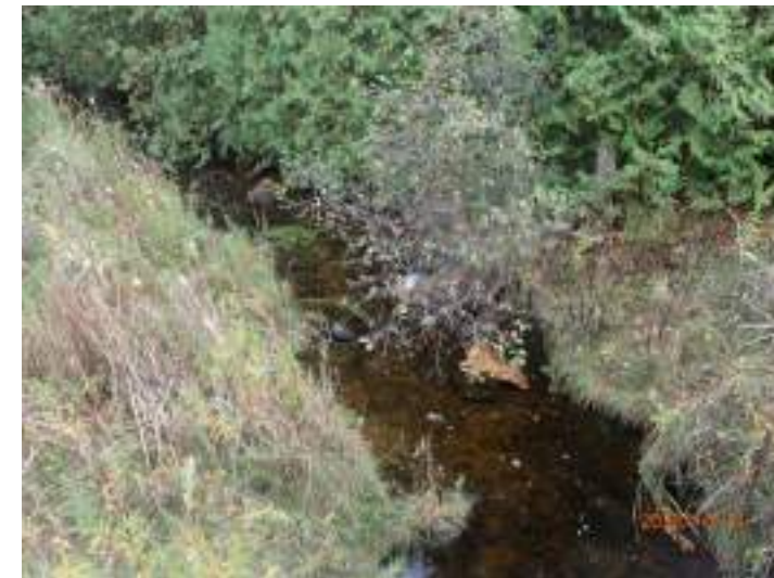
Plate 7: Biddy Creek Crossing 1 (C4) inlet, facing south (upstream).
