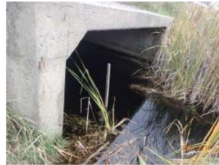
Plate 7: Bidy Creek Crossing 3 (C6) inlet, facing north (downstream).
