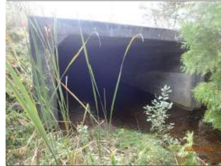
Plate 3: Bidy Creek Crossing 2 (C5) inlet, facing south (downstream).
