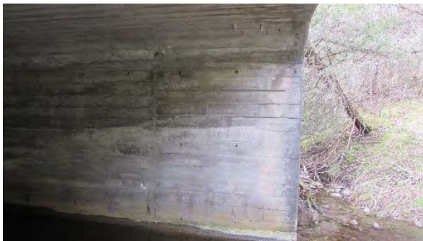
Culvert C473 North – High water level
