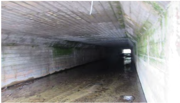
Culvert C472 North – Looking inside
