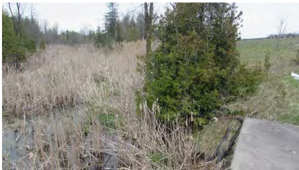
Culvert C471 North – Looking East
