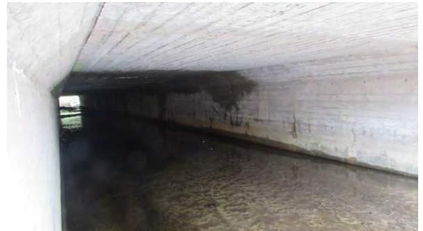
Culvert C473 South – Looking inside
