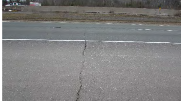
Culvert C474 North – Road
