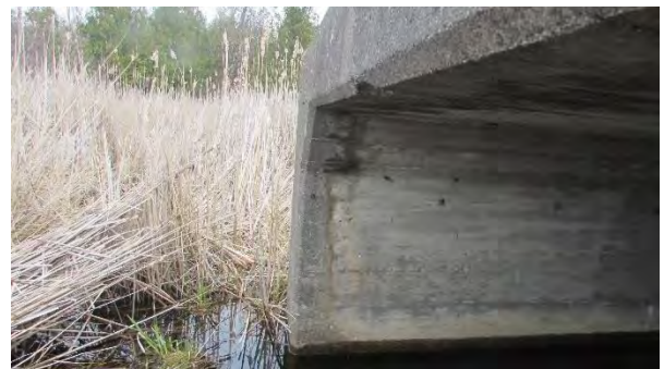
Culvert C474 North – High water level
