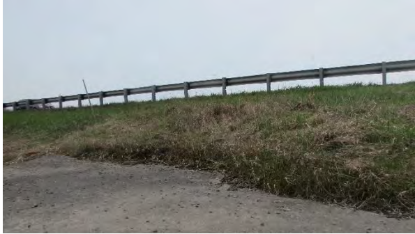
Culvert C474 North – Embankment
