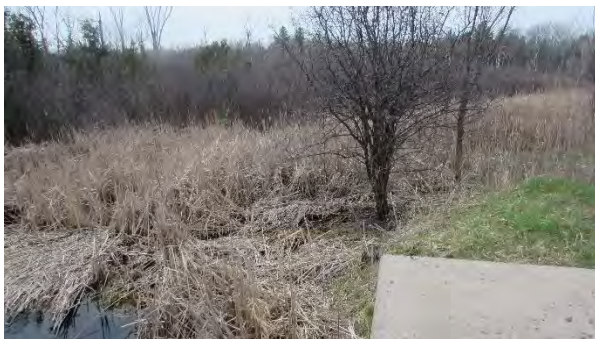
Culvert C474 South – Looking West
