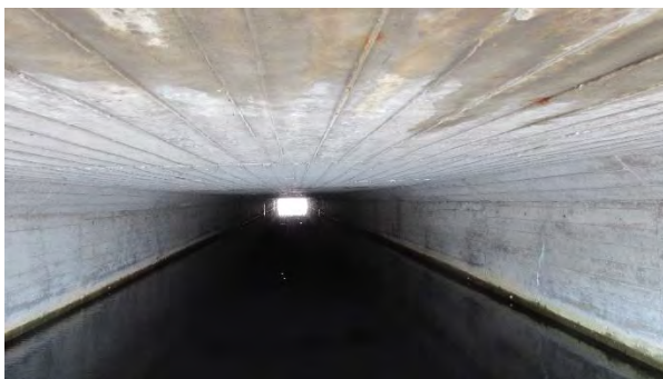
Culvert C474 South – Looking inside
