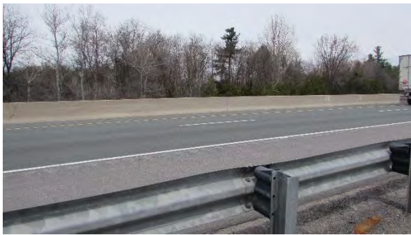
Culvert C473 South – Road
