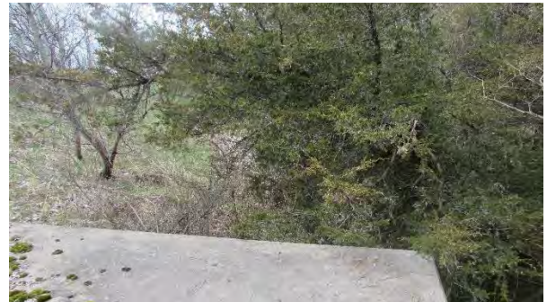
Culvert C473 North – Looking West
