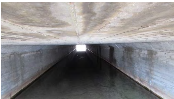
Culvert C41 South – Looking inside
