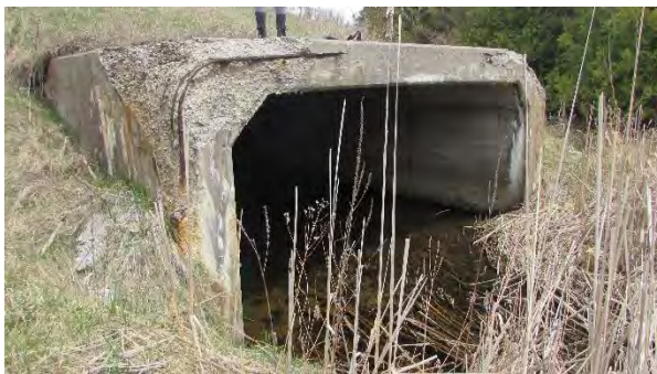
Culvert C473 South – Culvert end
