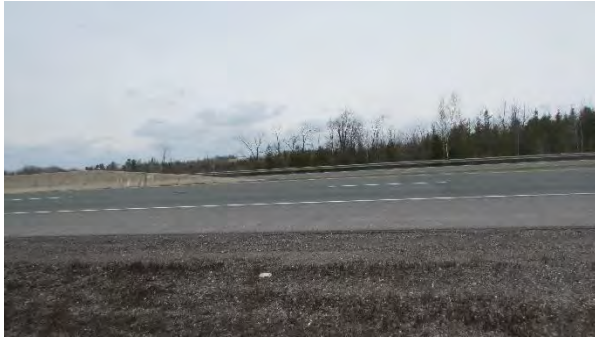
Culvert C474 South – Road
