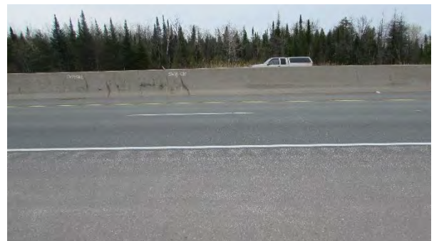
Culvert C471 North – Road
