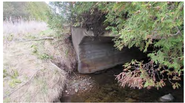
Culvert C472 North – Looking East
