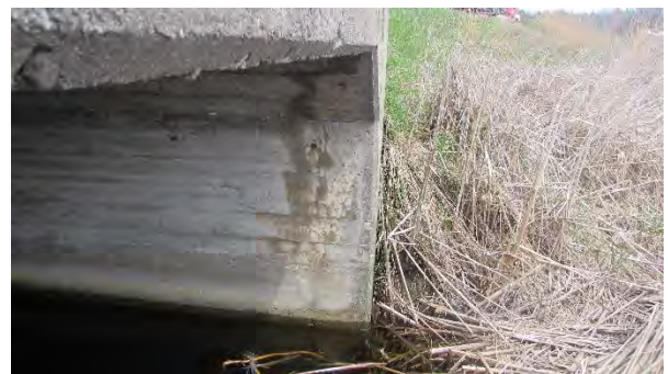
Culvert C474 South – High water level
