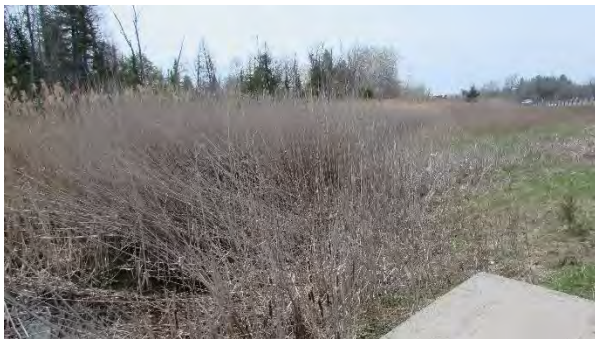
Culvert C471 South – Looking West
