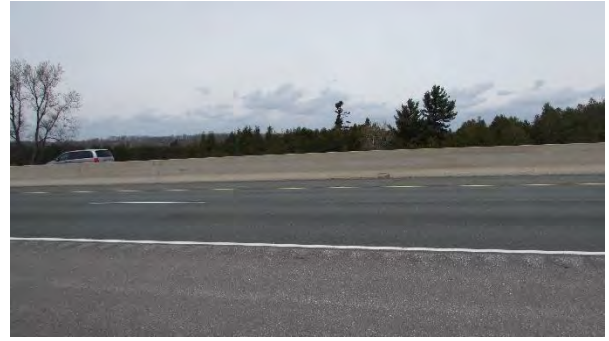
Culvert C472 South – Road
