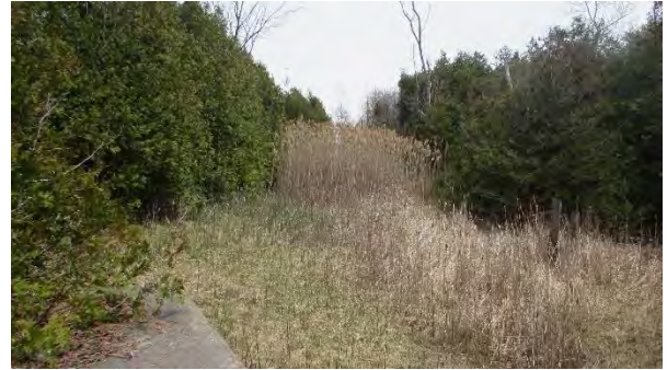
Culvert C472 South – Looking East
