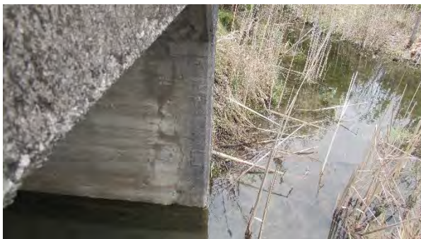
Culvert C471 North – High water level
