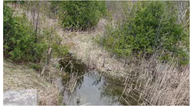
Culvert C471 North – Looking West
