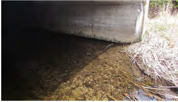
Culvert C473 South – High water level
