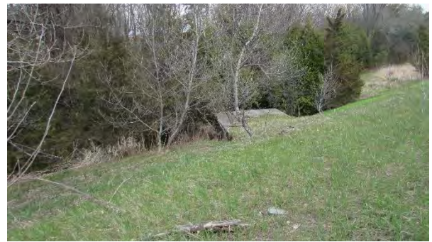
Culvert C473 North – Looking North
