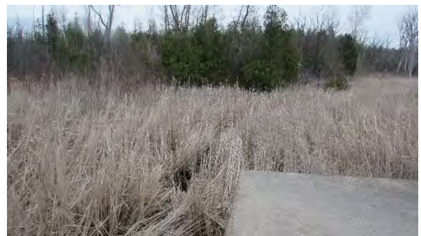
Culvert C474 North – Looking East
