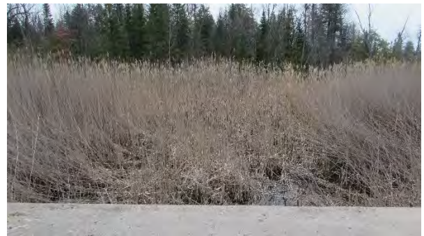
Culvert C471 South – Looking South
