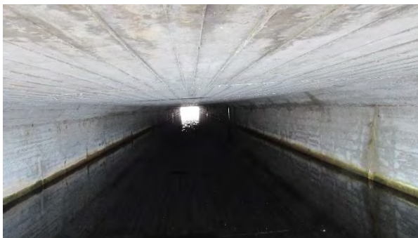
Culvert C474 North – Looking inside
