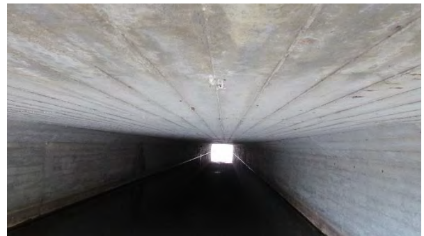
Culvert C471 North– Looking inside
