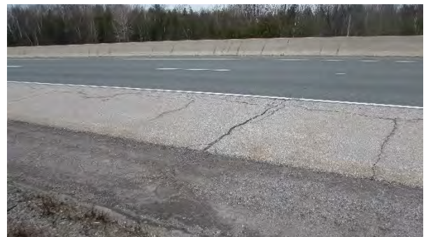
Culvert C471 South – Road
