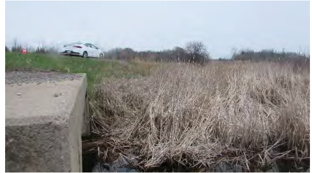
Culvert C474 South – Looking East
