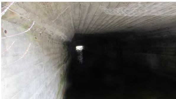
Culvert C472 South – Looking inside
