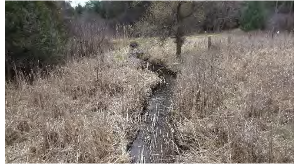
Culvert C473 South – Stream bank
