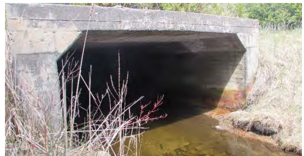
Culvert C472 South – Culvert end
