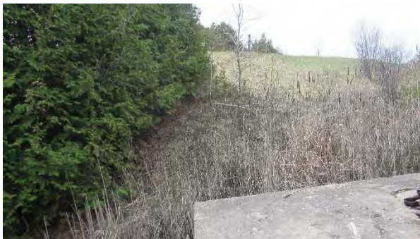
Culvert C472 South – Looking West
