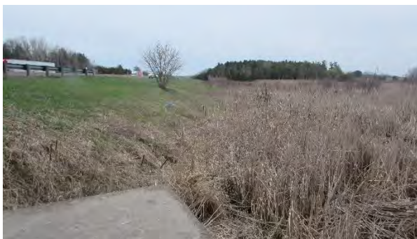
Culvert C474 North – Looking West
