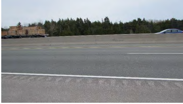
Culvert C472 North – Road
