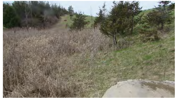
Culvert C473 South – Looking West
