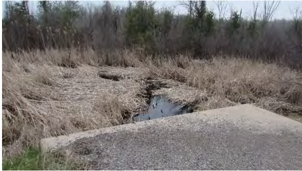
Culvert C474 South – Looking South
