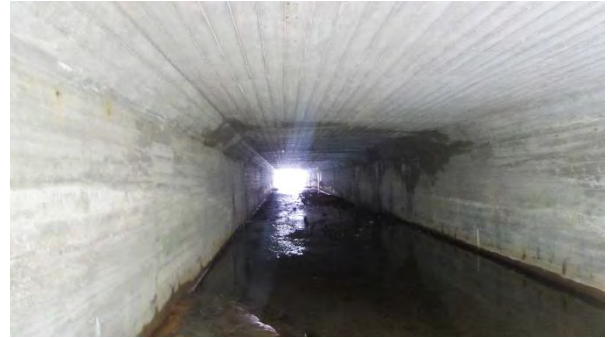
Culvert C473 North – Looking inside
