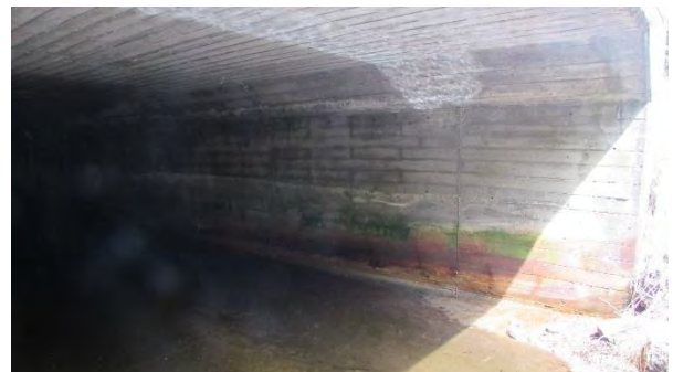
Culvert C472 South – High water level
