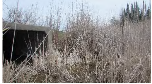
Culvert C471 South – Looking East
