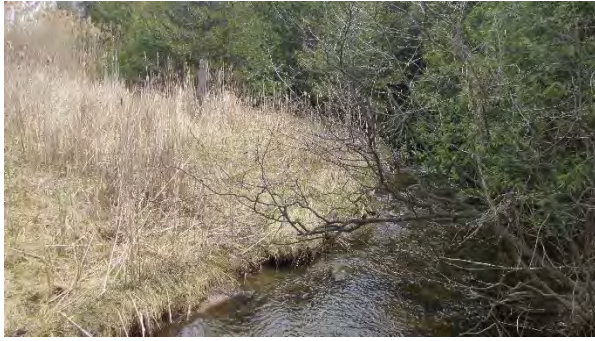
Culvert C472 South – Stream bank
