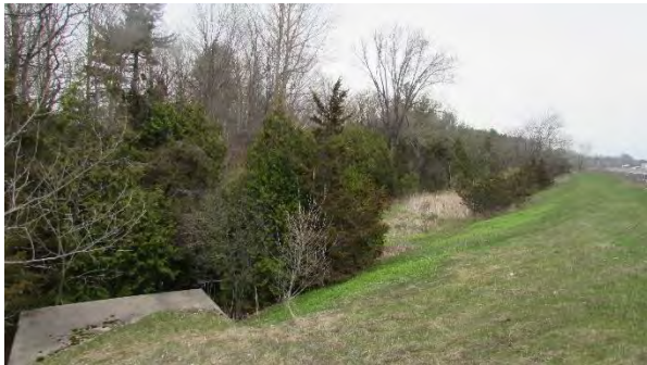
Culvert C473 North – Looking East
