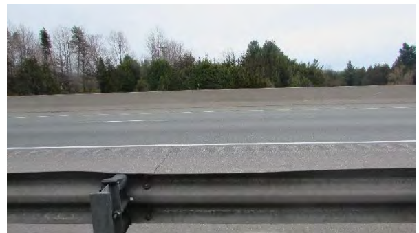
Culvert C473 North – Road
