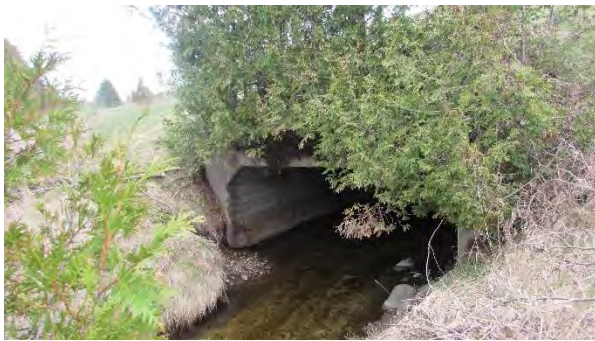
Culvert C472 North – Culvert end
