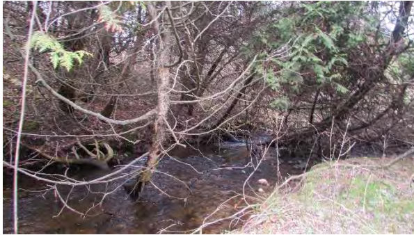
Culvert C473 North – Stream bank
