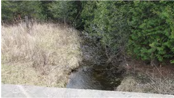
Culvert C472 South – Looking South
