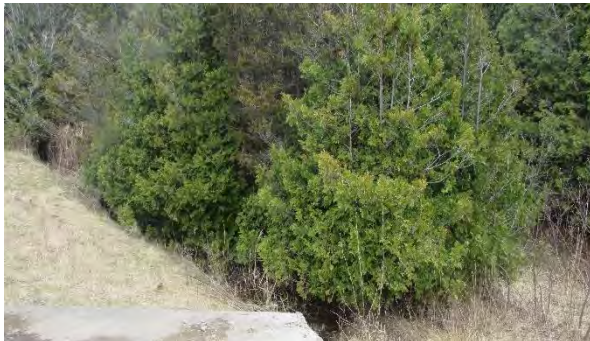
Culvert C473 South – Looking East
