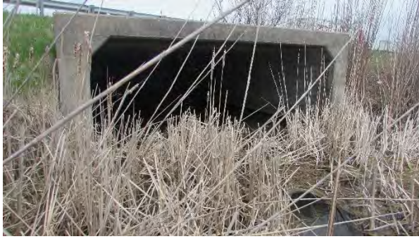
Culvert C471 South – Culvert end
