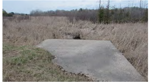
Culvert C474 North – Looking North
