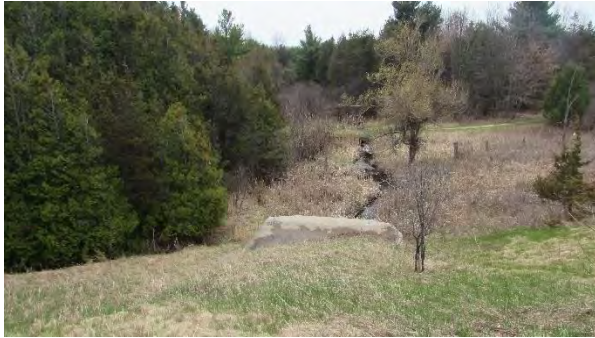
Culvert C473 South – Looking South
