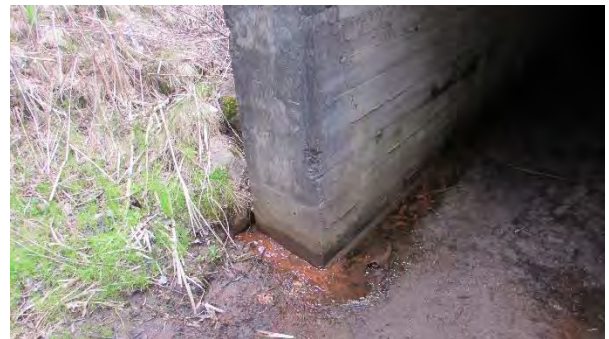
Culvert C473 North – East footing
