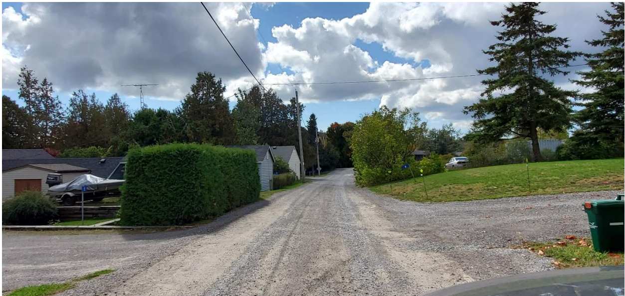
PHOTOGRAPH 10: NO MUNICIPAL SERVICING OBSERVED ON MCDONALD ROAD
