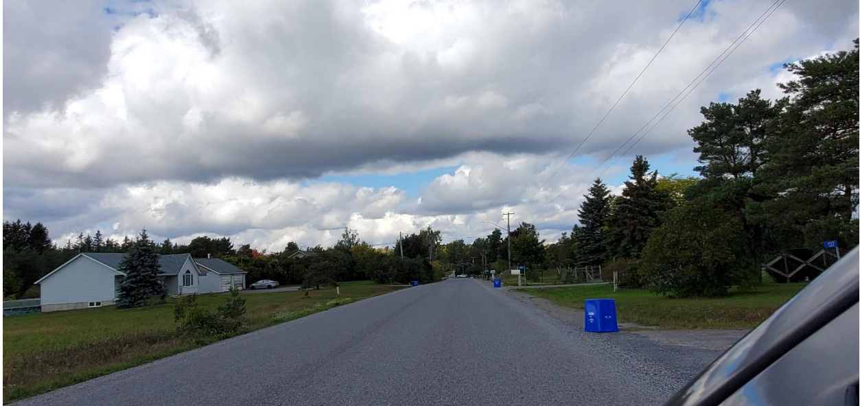
PHOTOGRAPH 11: NO MUNICIPAL SERVICING OBSERVED ON LAKE ROAD
