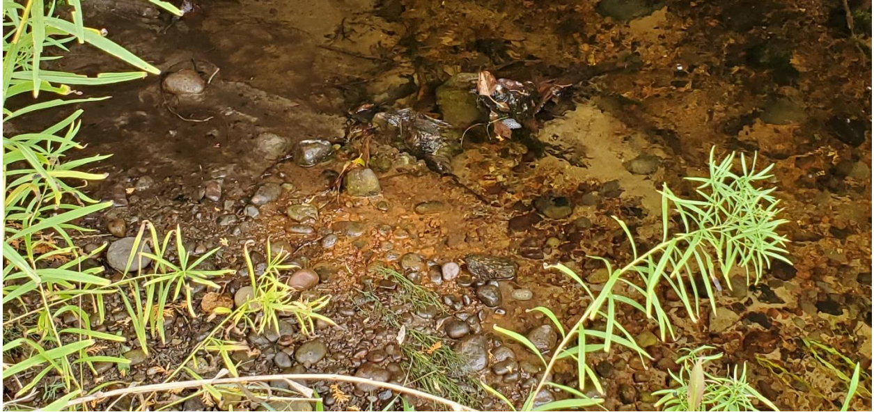
PHOTOGRAPH 13: IRON STAINING PRESENT AT CULVERT 21-472C, FACING NORTH
