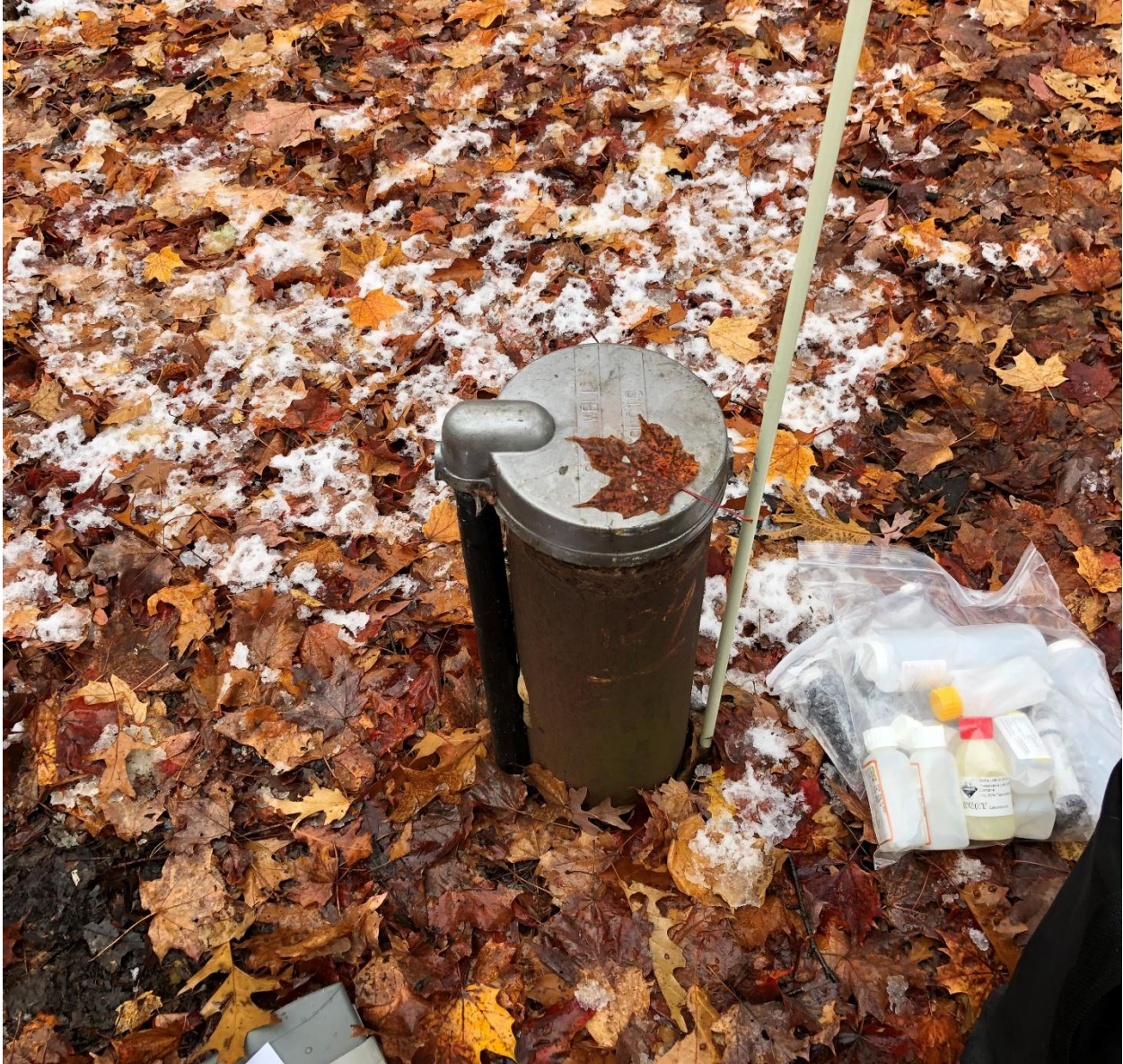
PHOTOGRAPH 21: DRILLED WELL AT 15791 TELEPHONE ROAD
