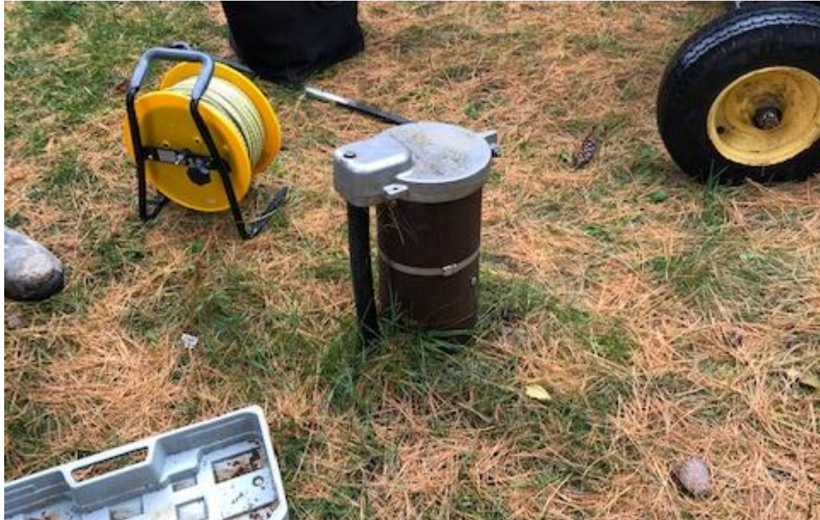
PHOTOGRAPH 18: DRILLED WELL AT 523 COUNTY ROAD 26
