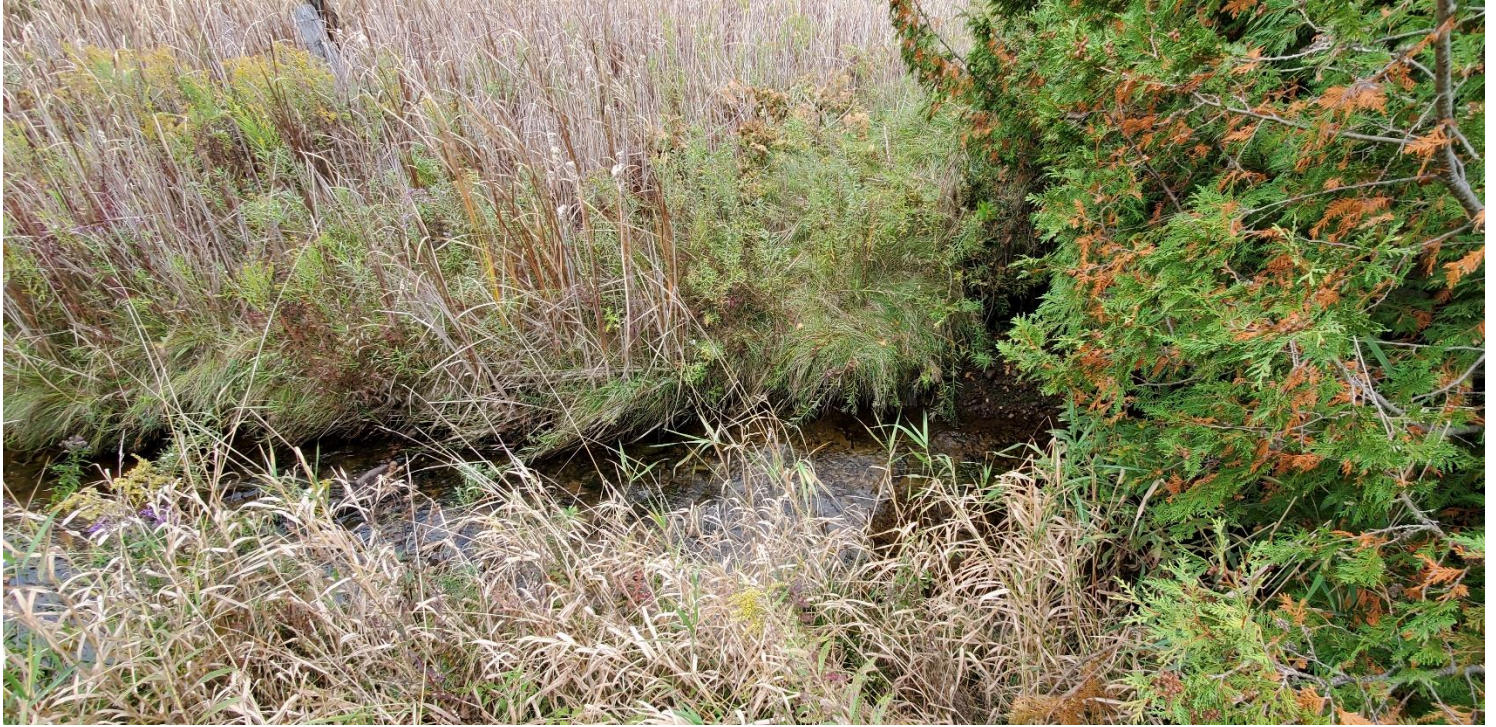
PHOTOGRAPH 7: WATERCOURSE AT CULVERT 21-472C, FACING WEST
