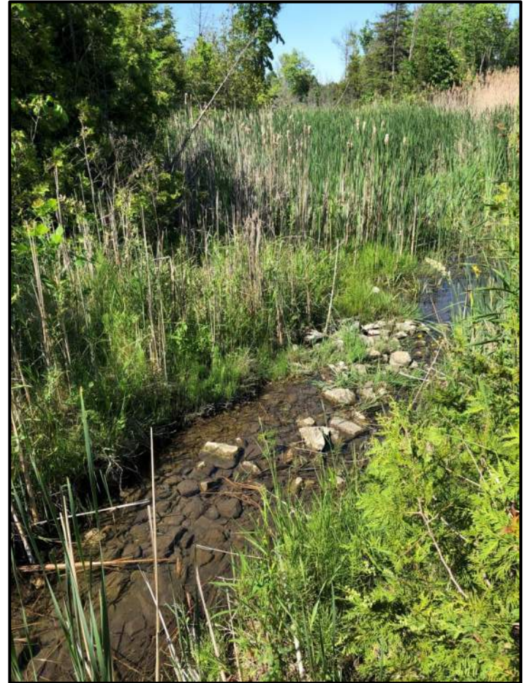
Looking downstream (North) from approximately 10m downstream of the culvert
