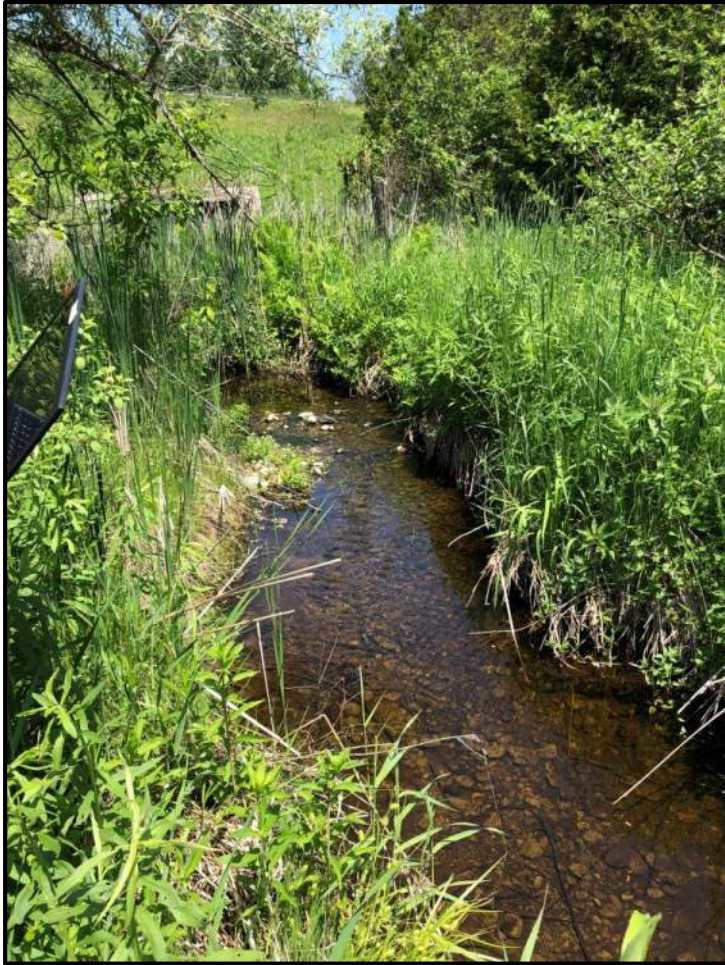
Looking upstream (North) from approximately 10m downstream of the culvert
