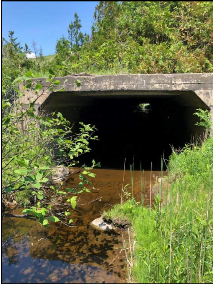
Looking downstream (North) from approximately 5m upstream of the culvert
