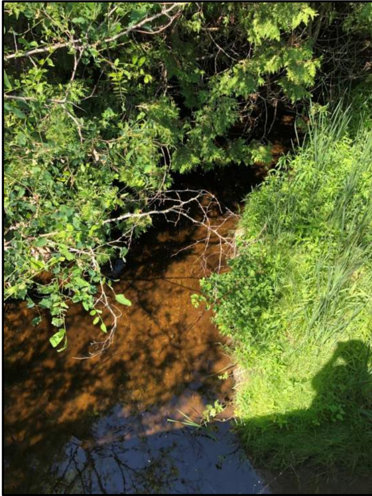
Looking downstream (North) from the culvert
