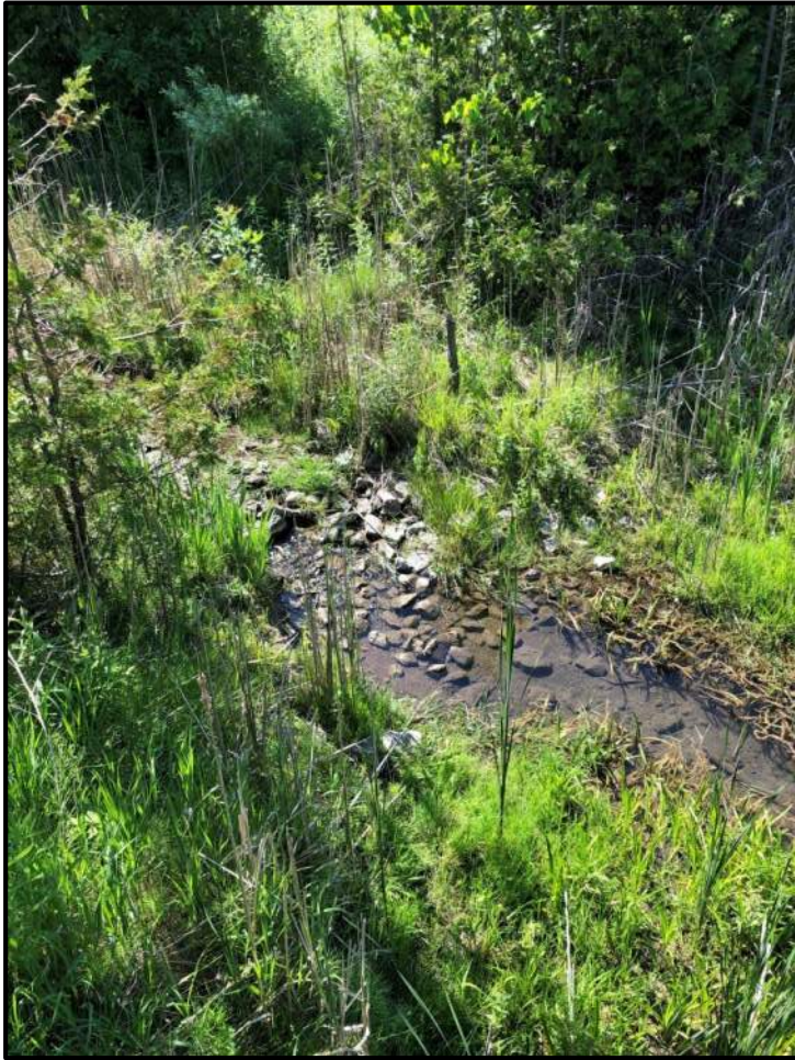
Looking upstream (South) from the culvert
