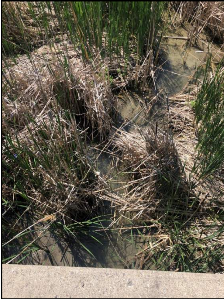
Looking upstream (South) from the culvert
