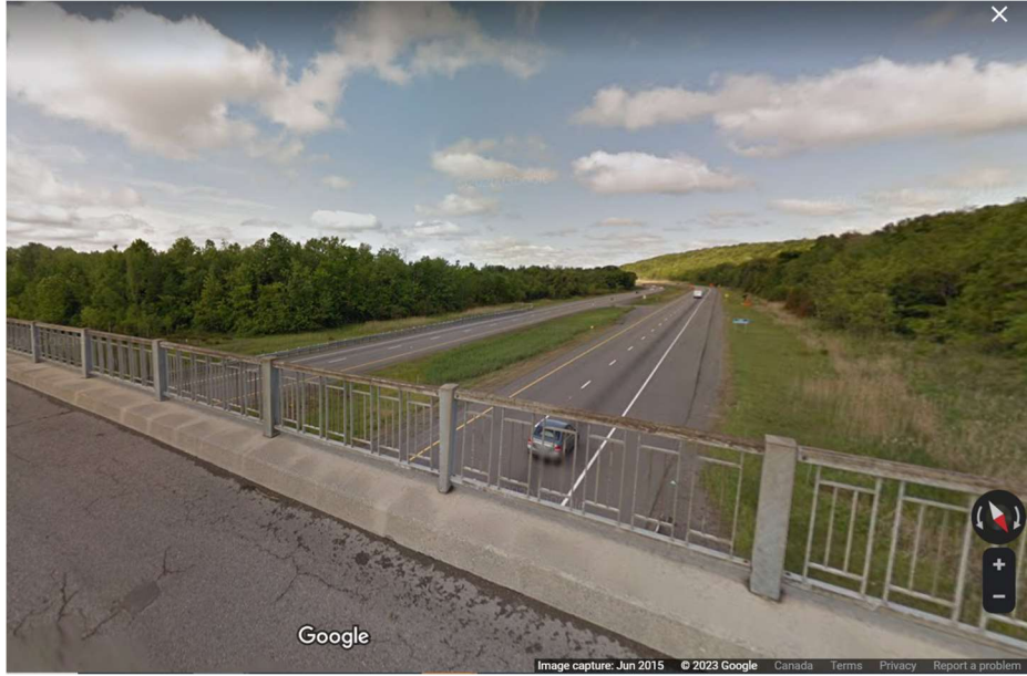
Figure 8 - View of Highway 401 from Christiani Rd. bridge, looking west
