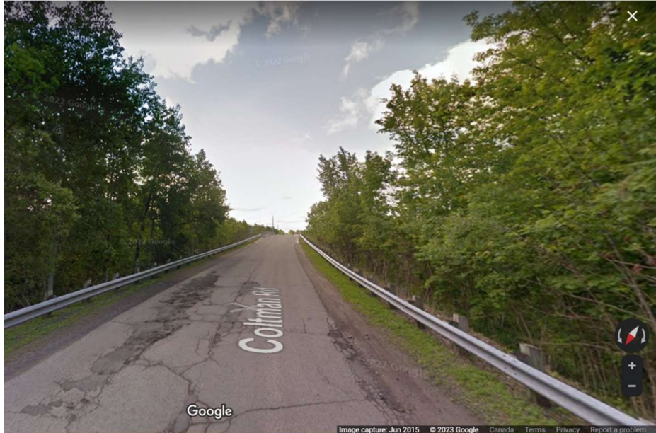
Figure 9 - View of Christiania/ Coltman bridge approach over Hwy 401, looking south
