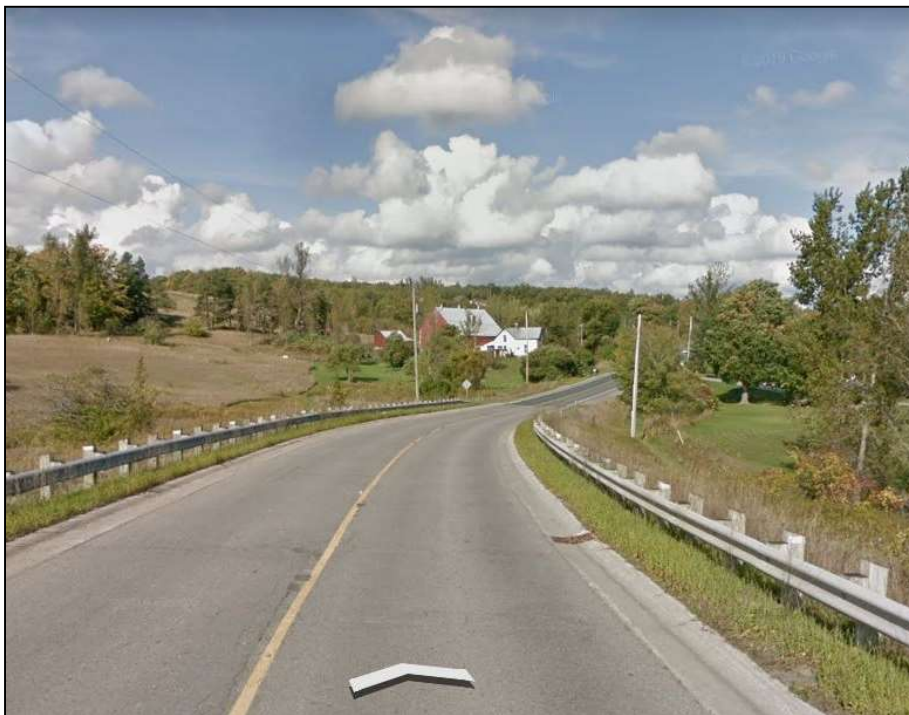
Figure 3 - County Road 26 north of Highway 401, looking north
