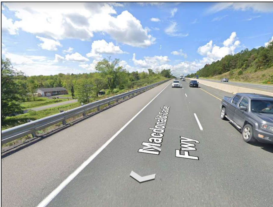
Figure 5 - Eastbound lane of Highway 401, looking south west
