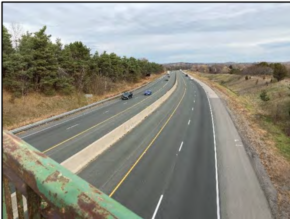
Image 13: Artificially cut slope along Highway 401 right-of-way. Facing northeast.
