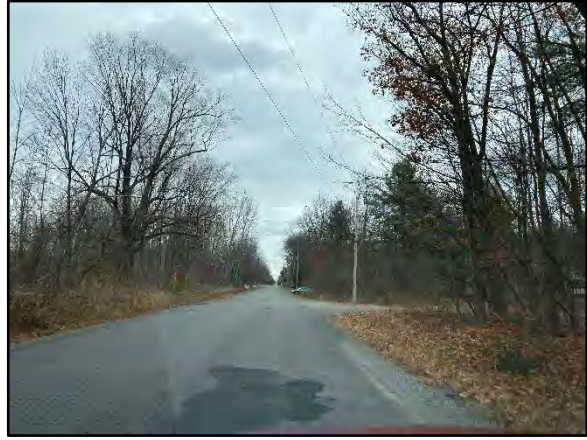
Image 28: Field Conditions along Telephone Road. Facing east.
