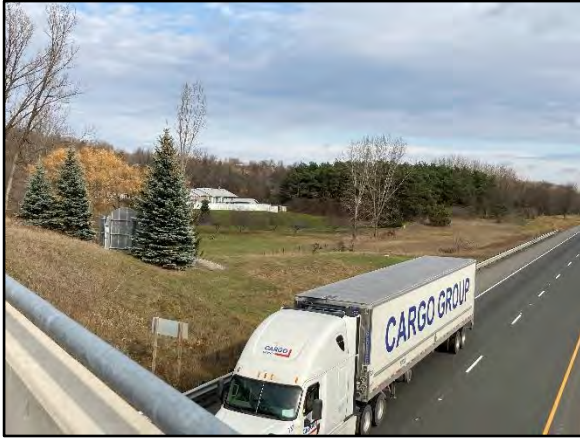
Image 15: Overpass berm. Facing northeast.
