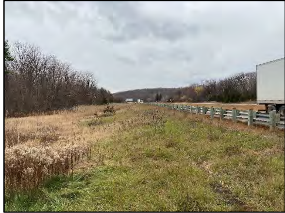
Image 6: Field conditions along Highway 401 right-of-way. Facing west.
