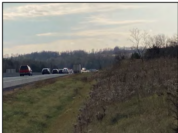
Image 10: Ditching and artificial berm along Highway 401 right-of-way. Facing southwest.
