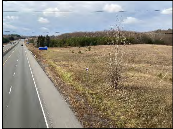
Image 8: Ditching and drainage along Highway 401 right-of-way. Facing west.
