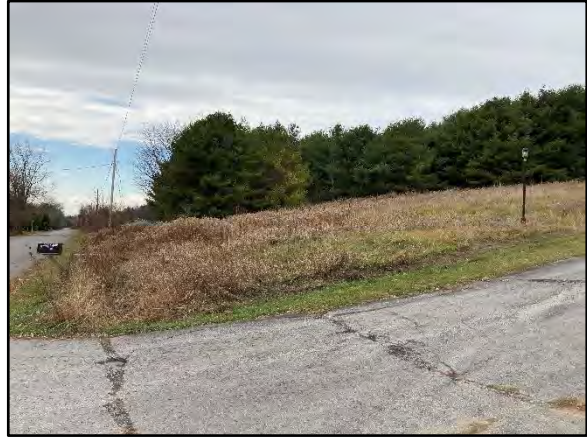
Image 32: Area of steep slope (>20°) along Crandall Road. Facing northwest.
