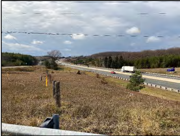
Image 7: Disturbance along Highway 401 right-of-way (Note yellow gas line marker along fence line). Facing west.
