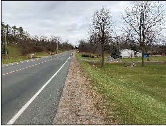
Image 27: Manicured lawn, residences, and ditching along County Road 26 right-of-way. Facing northeast.
