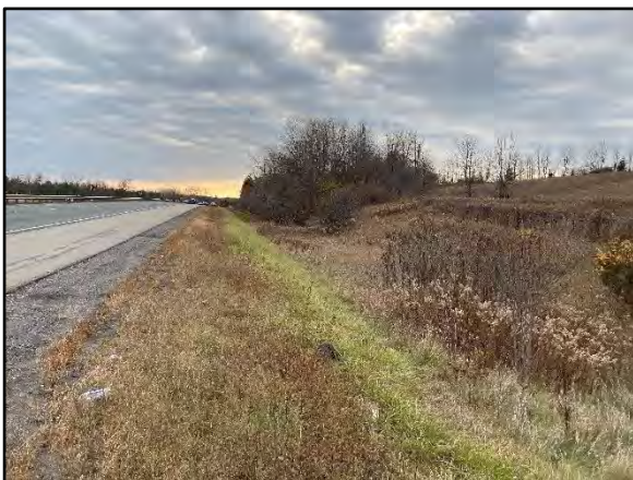
Image 9: Ditching and drainage along Highway 401 right-of-way. Facing southwest.
