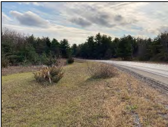
Image 25: Field conditions along County Road 26. Facing southeast.
