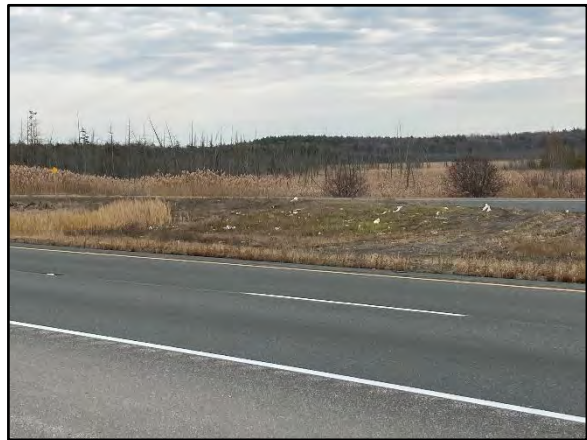
Image 4: Ditched median along Highway 401. Facing southeast.
