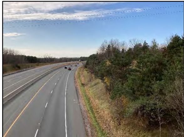
Image 14: Artificially cut slope along Highway 401 right-of-way. Facing southwest.
