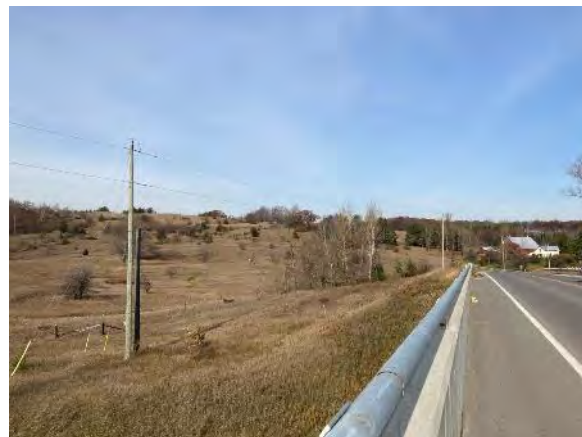
Image 37: View of County Road 26 looking north from Highway 401 underpass
