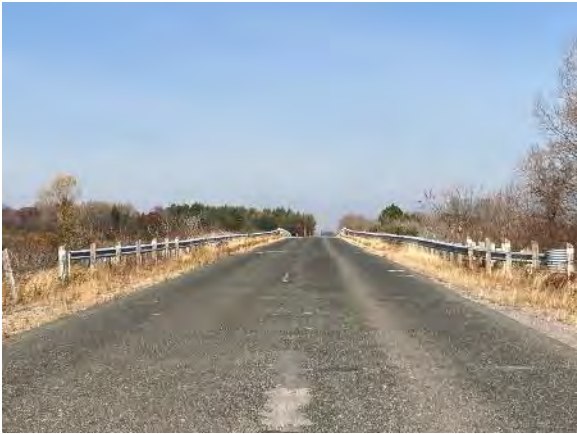
Image 10: View of Durham Road looking north to Herley Road Underpass over Highway 401
