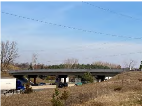
Image 38: View of County Road 26 Underpass, looking east
