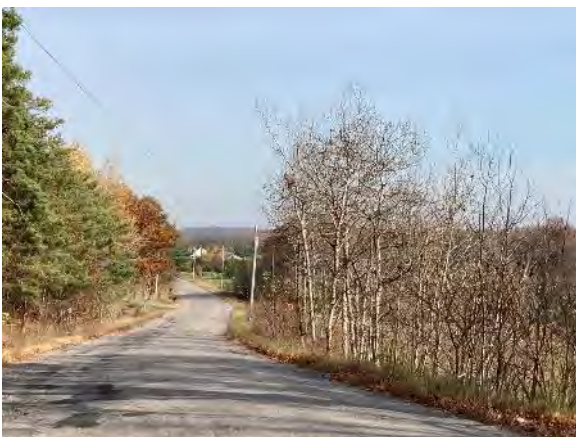
Image 16: Crandall Road looking east from east of Honey Road
