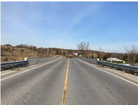
Image 36: View of County Road 26 Underpass, looking north
