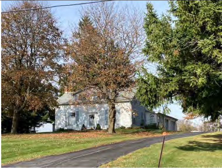
View of the farmhouse at 15064 Telephone Road, looking north
