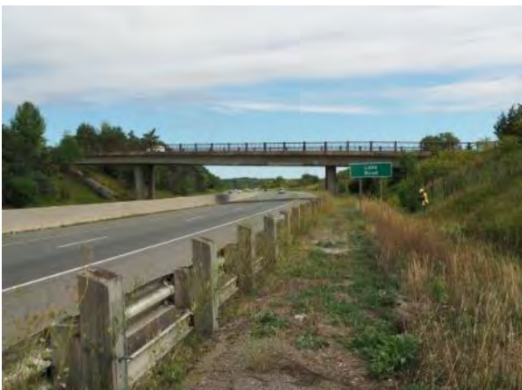
Image 24: View of Lake Road Underpass, looking east from Highway 401
