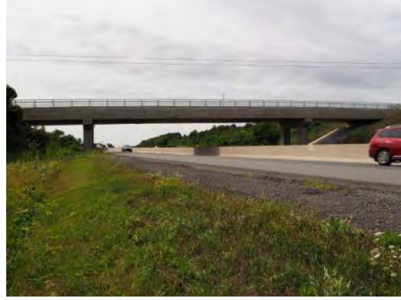
Image 13: View of Herley Road Underpass looking west from Highway 401
