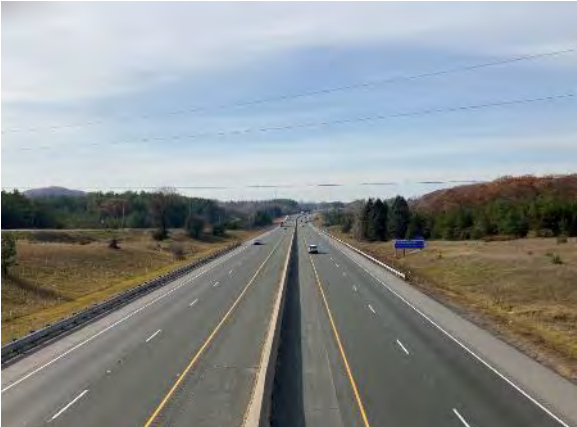
Image 6: View of Highway 401 from County Road 26 Underpass, looking west
