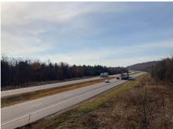
Image 7: View of Highway 401 from Christiani Road Underpass, looking west
