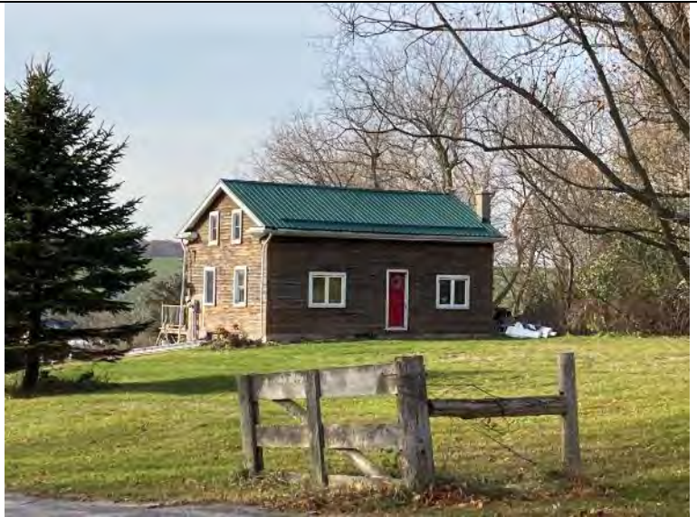
View to 148 Samis Road looking west
