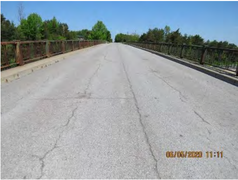
Figure 2: Bridge Along Roadway
