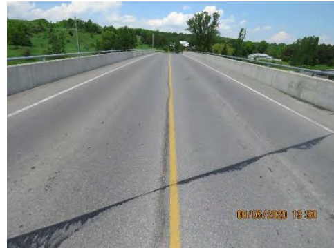
Figure 2: Bridge Along Roadway
