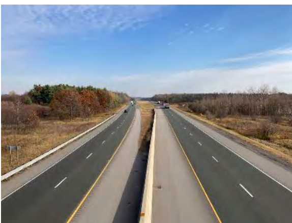
Image 1: View of Highway 401 from Herley Road Underpass, looking east
