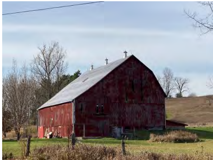
View to the property at 638 County Road 26 (above) and to the property's barn (below), looking north
