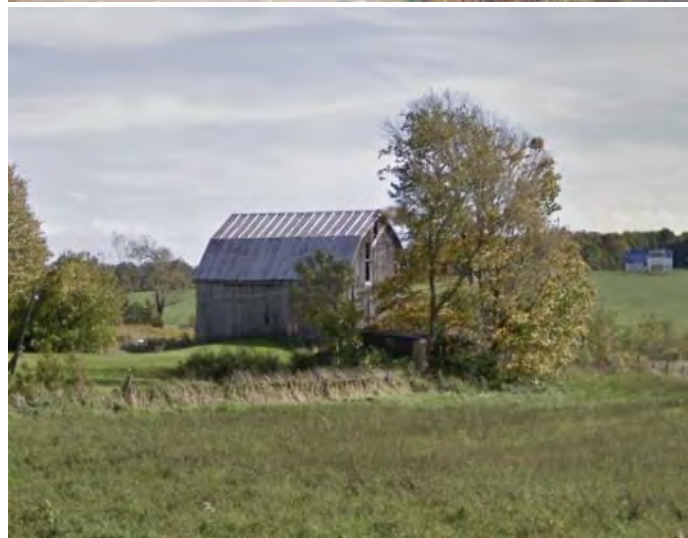
View to the farmhouse at 15154 Telephone Road (above) and the barn (below), looking south
