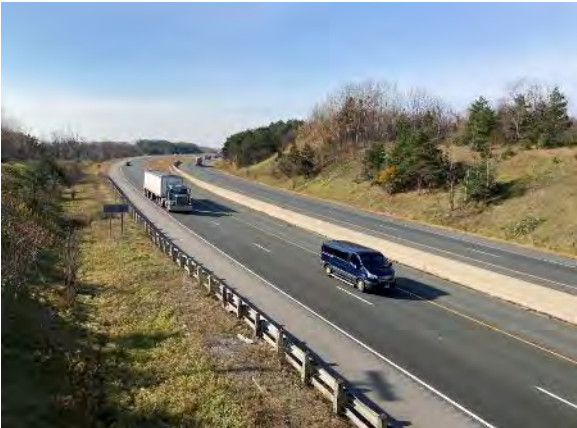
Image 4: View of Highway 401 from Lake Road Underpass, looking west
