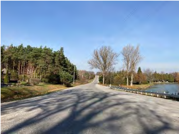
Image 20: View of Lake Road looking north from Pine Tree Lane to Highway 401
