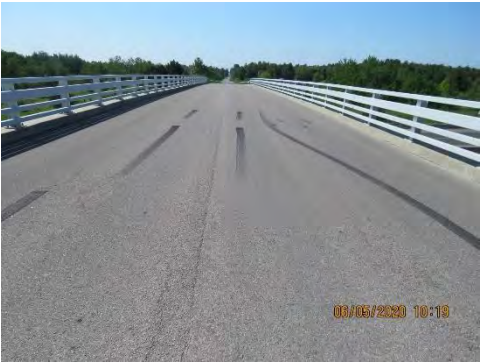
Figure 2: Bridge Along Roadway
