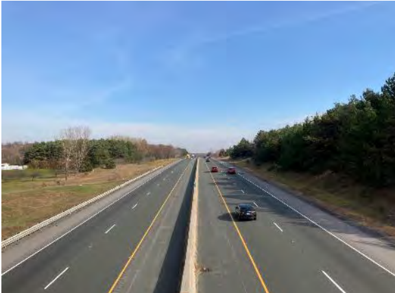
Image 5: View of Highway 401 from County Road 26 Underpass, looking east
