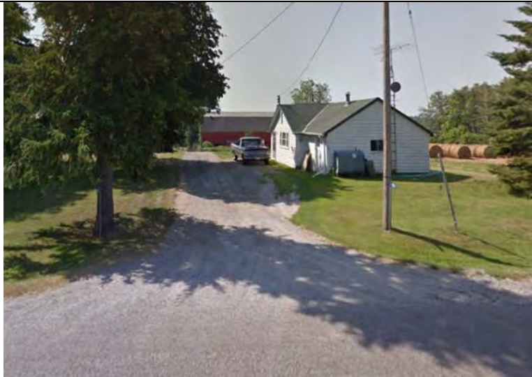
View of the property at 13711 Telephone Road looking south
