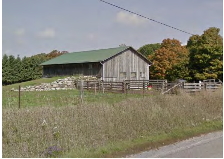
View of the barn at 14764 Little Lake Road, looking northeast
