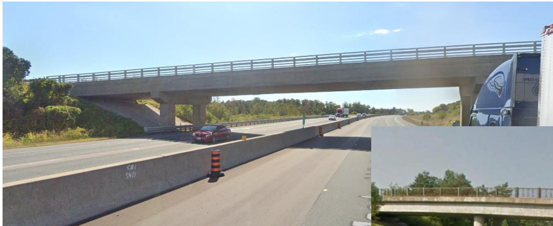
Herley Road Underpass
